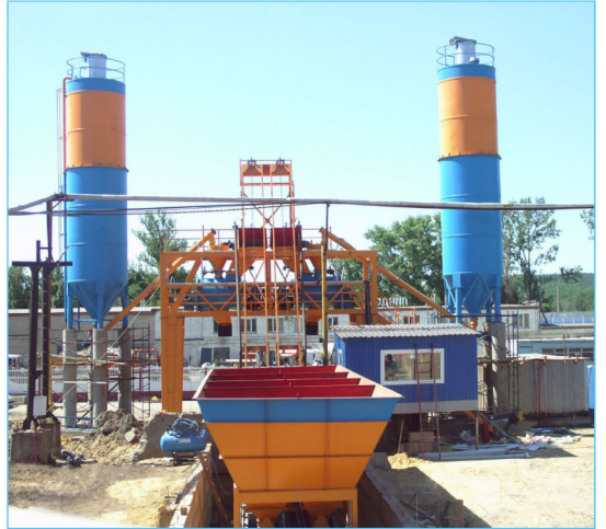
60+60m 3 /h kovalı sabit beton santrali
